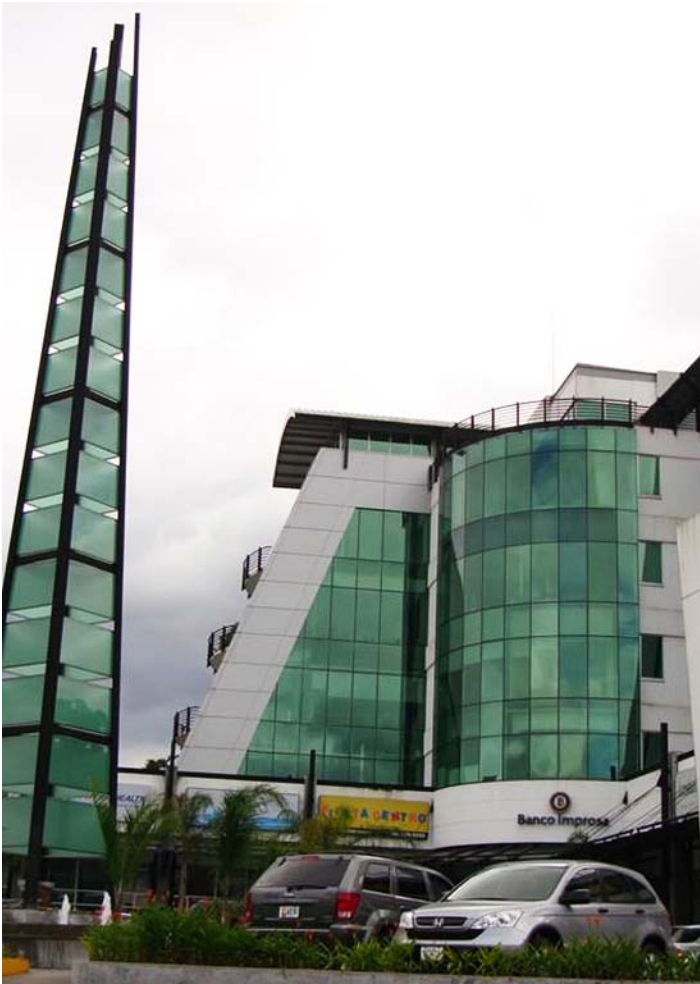
Office Building in Costa Rica
